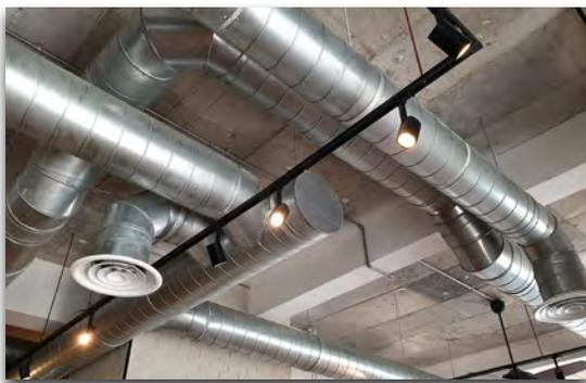
Improved ventilation can be achieved by increasing the outdoor air supply through the HVAC system or by supplementing with passive outdoor ventilation from open windows or doors. Buildings can also run the HVAC 24/7 to further increase the amount of outdoor air brought indoors. While constantly running HVAC can improve indoor air quality, consider using clean energy sources so that outdoor air is not adversely affected by pollution caused by increased use and fossil fuels.<sup>2</sup>
